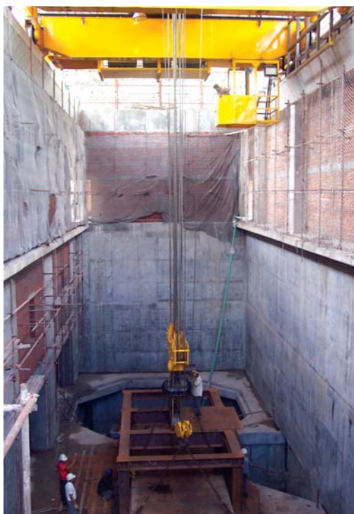
Work in progress inside the Powerhouse
