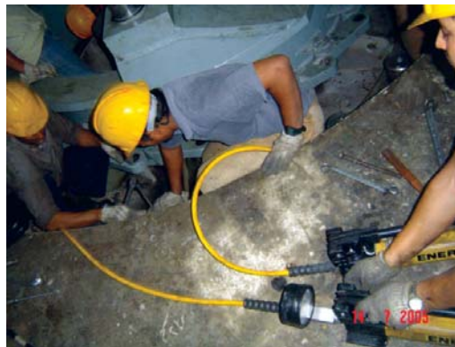
Repair of turbine of KG 'A' HES
