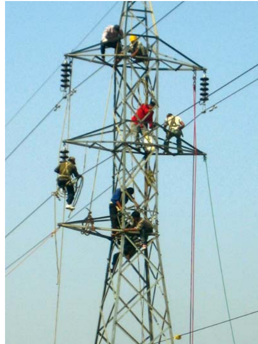
Maintenance of 66 kV Trishuli - Balaju transmission line.
