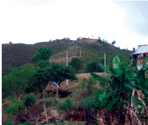
Eight Power Project - Distribution line construction, Dhading.
