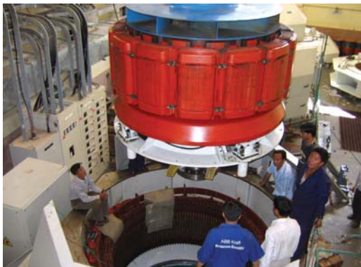
Maintenance of turbine runner of Modi Khola Hydro Power Station
