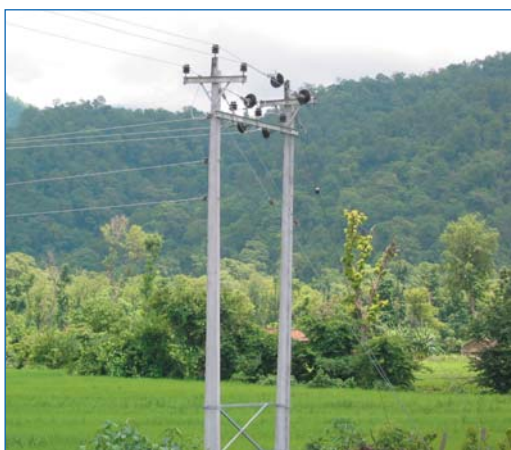
Sindhu Dolakha Distribution Line Extension Project
