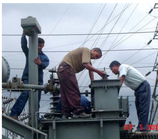
Transformer repair of Siuchatar Substation
